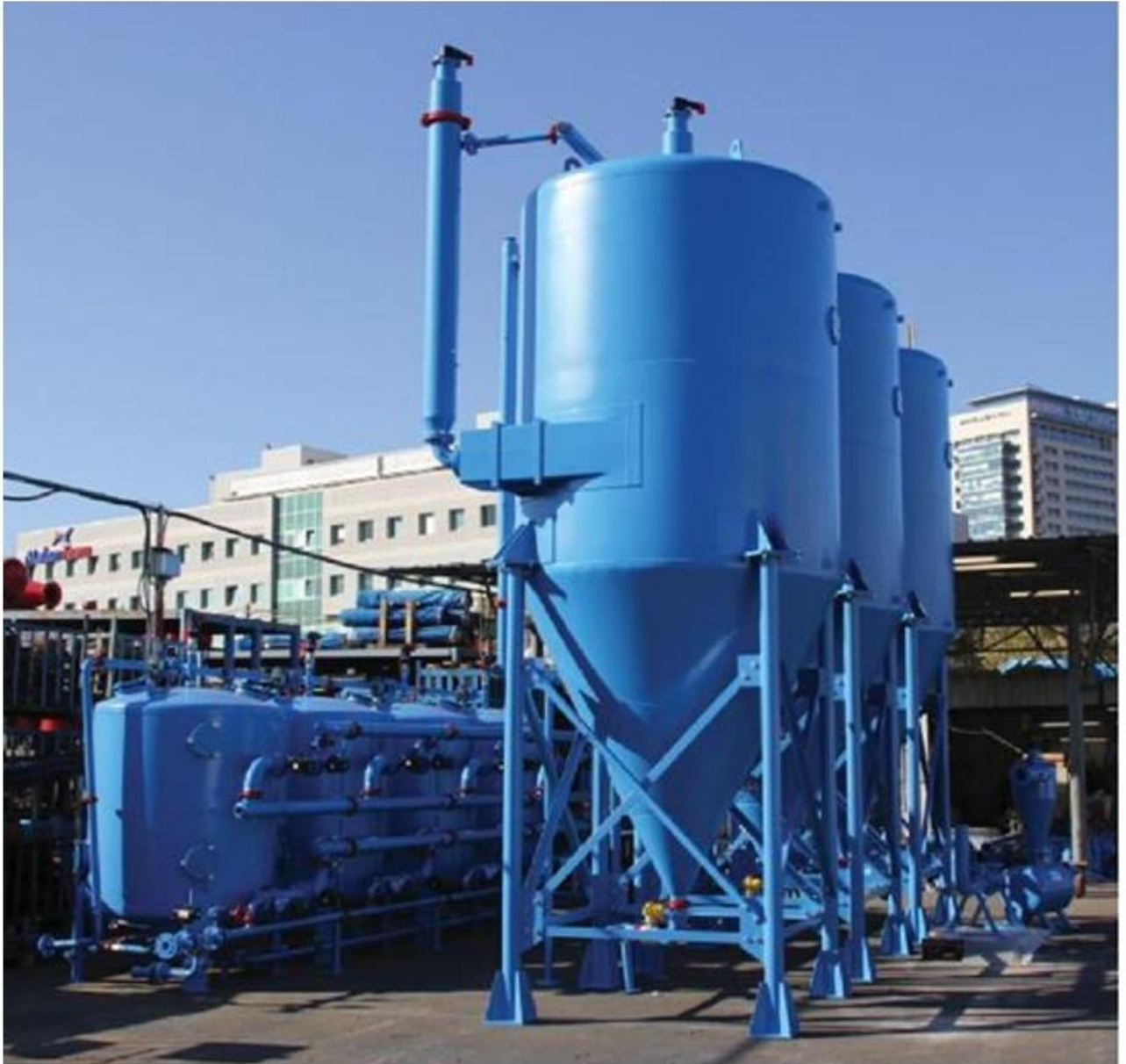
THE FIRST WASTEWATER TREATMENT SYSTEM CONVERTED TO DRINKING WATER IN VIETNAM AT YEN PHU WATER PLANT CAPACITY: 2,400 m 3 /day (YEAR 2014).
